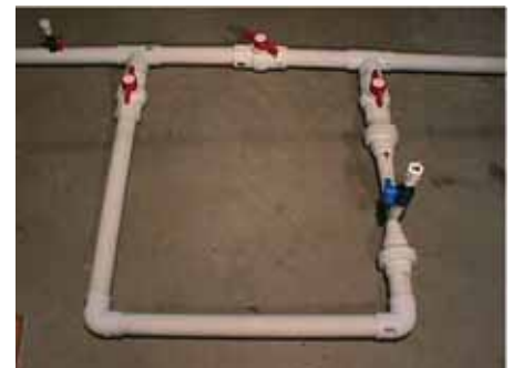
Figure 19D - Below Grade
