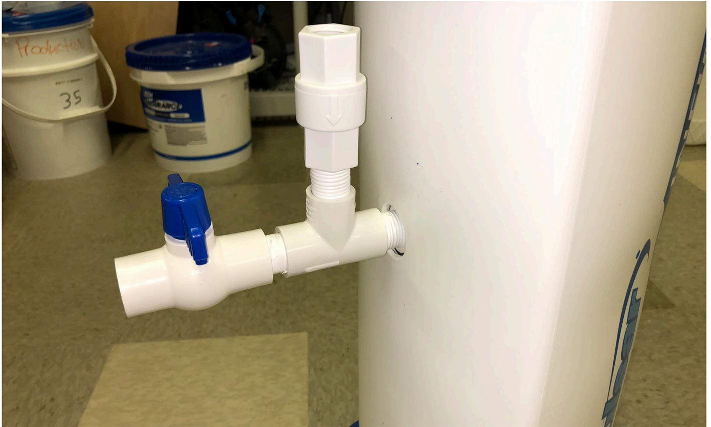
**STEP 2** – Complete the drain/vent by putting the ball valve at the end of the Tee to contain the flow during normal operation of the feeder.
