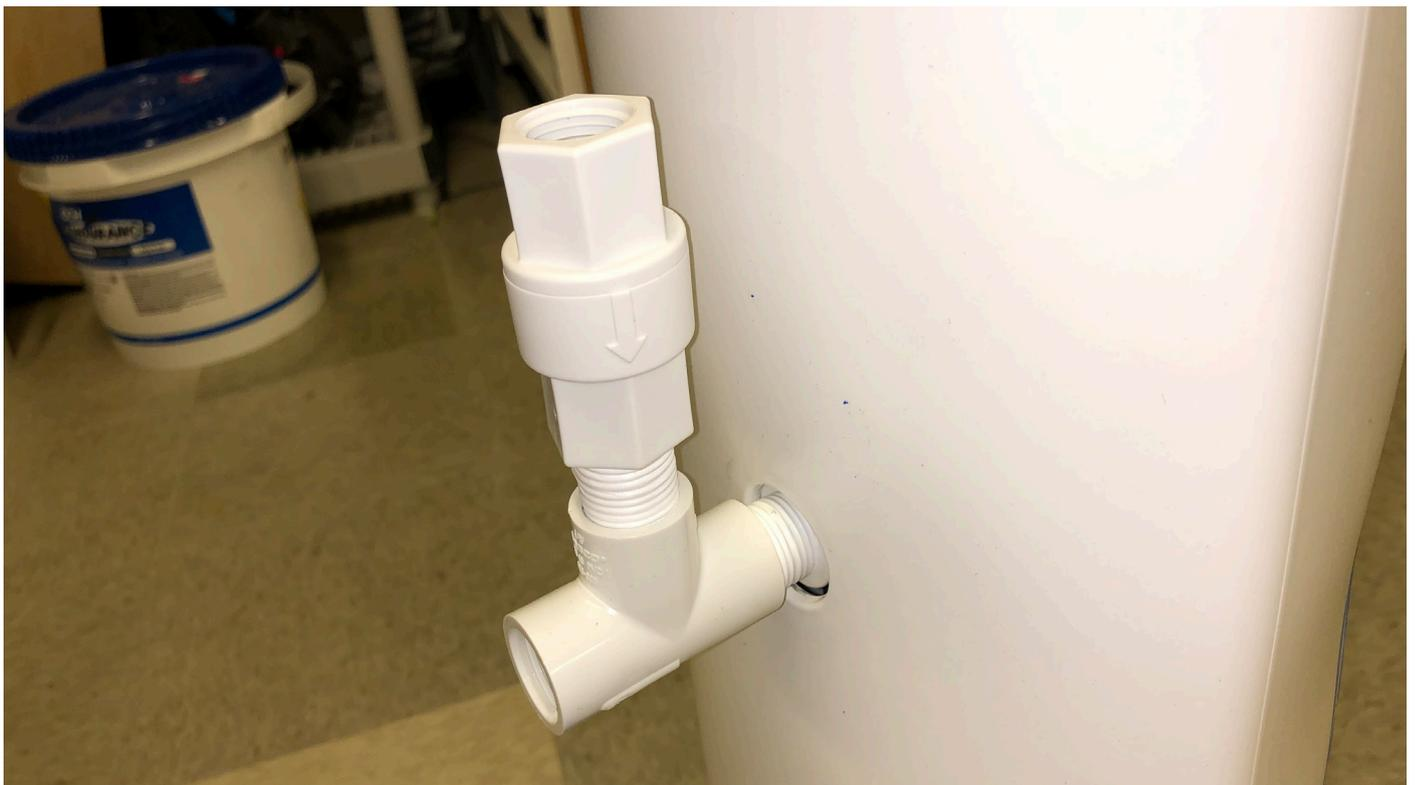
**STEP 1** – For air venting capabilities, install the 1/2" check valve with the arrow pointing down using the other 1/2" tee and remaining nipples
